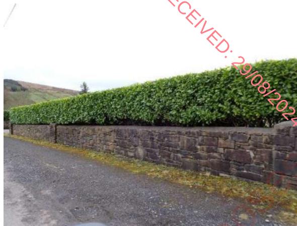
Plate 6.12 Man-made stone wall present at parking bay 5 (PB5).
