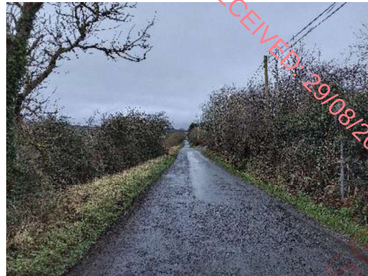
Plate 6.16b UEEC route, at structure 8.
