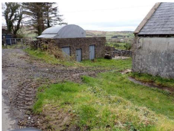
Plate 6.11 Man-made structures present at parking bay 2 (PB2).
