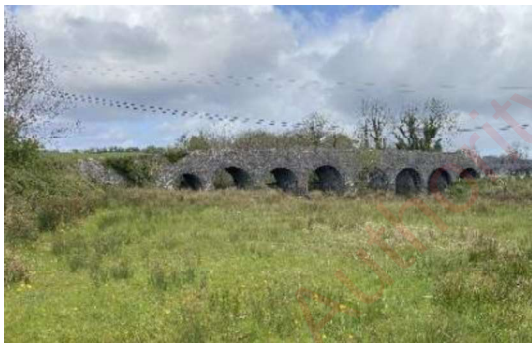
Plate 6.48c Tonrehown Bridge crossing the Cloonaghmore River.
