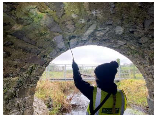
Plate 6.48f Inspection of bridge for evidence of roosting bats using endoscope.
