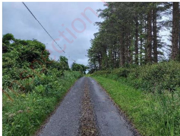
Plate 6.14 Existing tarmacadam road proposed for site access.
