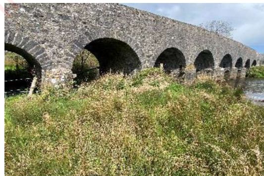
Plate 6.48d Tonrehown Bridge crossing the Cloonaghmore River.
